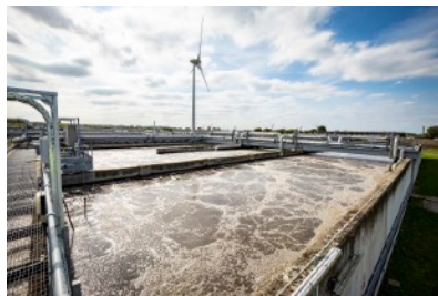
Aeration lane in a sewage treatment works. Image: Thames Water
